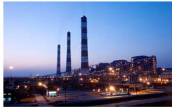
NTPC Sipat (3x660MW)
