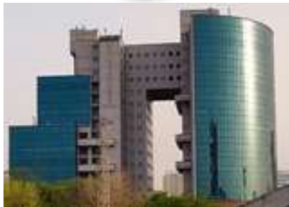
New Head Office at Signature Tower
